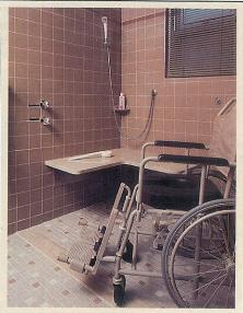
excessive transfers. The 18-inch-high toilet stands taller than usual. A roll-in shower features a "lead pan" drain, so a lip to catch water — which would act as a barrier — is unnecessary. The shower head can be either hand held or wall hung and contains water pressure and temperature controls. The marble bathing seat adds luxury to a basic and practical design. ELIZABETH GAYNOR
