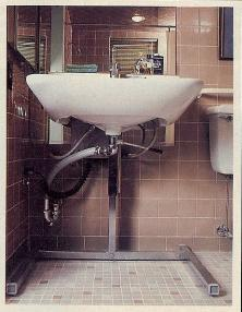
stainless-steel shelf rises (above, center) and descends (above, left) in response to its user's needs. An under-sink mounting stand permits wheelchair pull up, and flexible conduit hosing substitutes for fixed plumbing to make sink movement possible.
